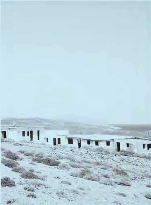
← Remnants from the barite washing facility.
