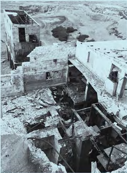
← Abandoned housing near the mines.
