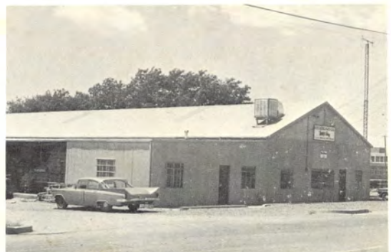
FARMINGTON, NEW MEXICO, district office and warehouse. Well built, well lighted warehouses such as this provide employees with best possible working conditions and insure maximum protection for stored products.
